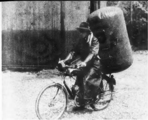
Lightweight gas bag on cyclist's back provides him with cheap source of power. But not only is it inexpensive — more important, it's available!
